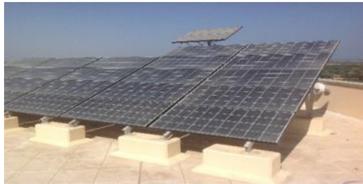
Figure 4: Example of Dust Accumulation on Solar Panels
