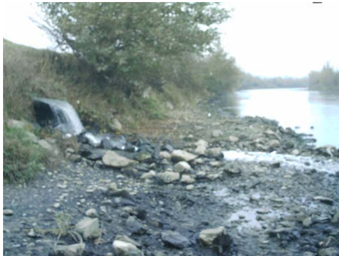
Figure 3. Wastewater discharge in Jiu River
