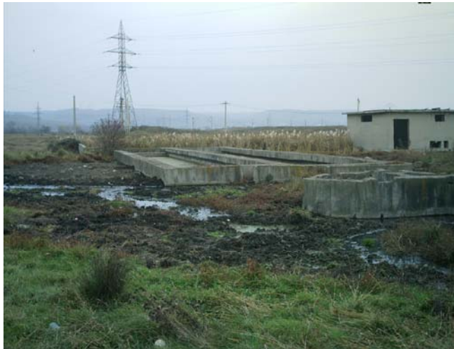
Figure 2. Wastewater Treatment Plant in Rovinari
