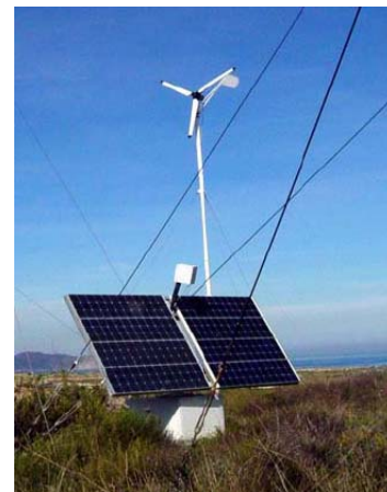
Figure 4. The small hybrid system
