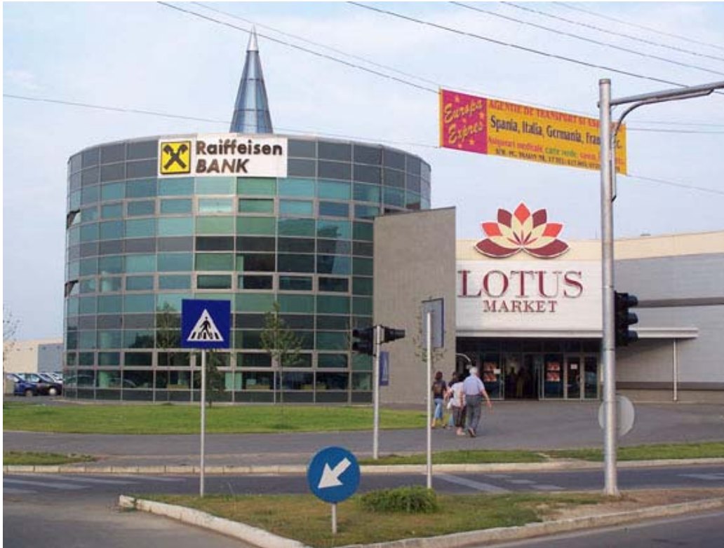
Figure .1. Raiffeisen bank headquarters in the Lotus Market complex.
