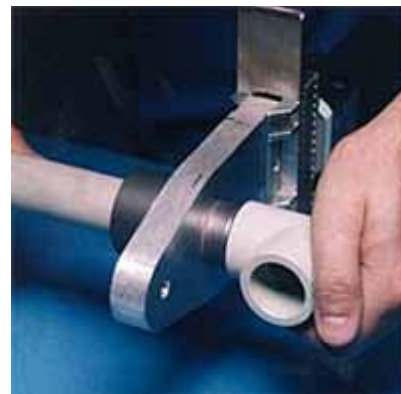
Fig.4. Socket fusion welding
