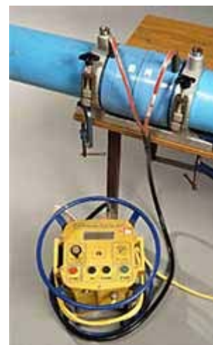
Fig.5. Electrofusion welding
