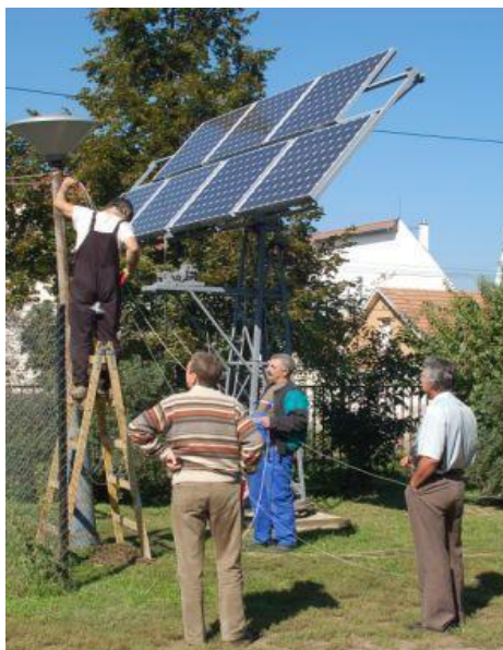
Figure 1. Last phases of the installation
