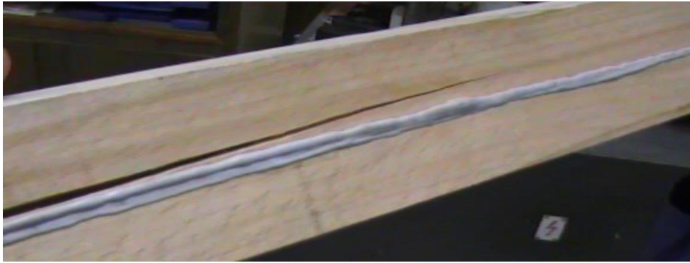
Fig. 1 Tension failure of a reinforced wood beam with one CFRP sheet
