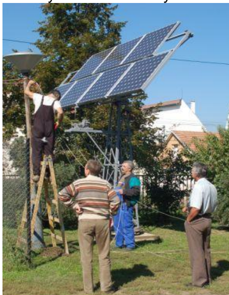
Figure 1. Last phases of the installation
