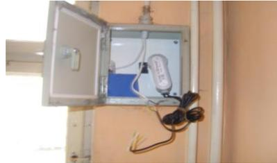
**Figure 5. Replacing electronic reader CF M-BUS COMBI network radio module Sensus ((S)) cout-P2 in block staircase [1]**
