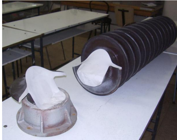
Fig. 2.1. Ceramic Insulator broken from the metallic bottom support
