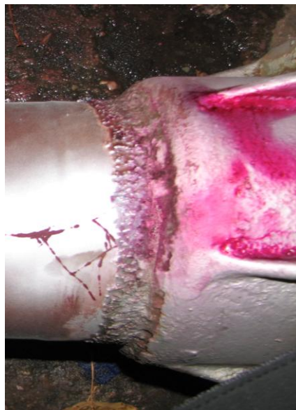
Fig.4.6. Cracks and boundary cement destruction.
