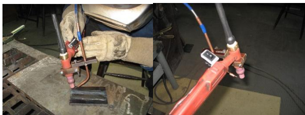
Fig. 2. Preparing WIG welding head for mechanized feed based welding
