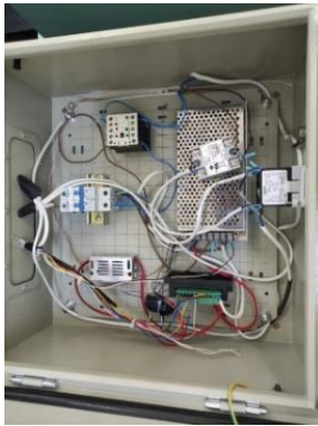
Figure 12 Control panel mounting
